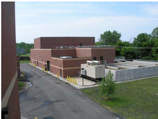
Figure 1.4. Mankato Water Reclamation Facility
