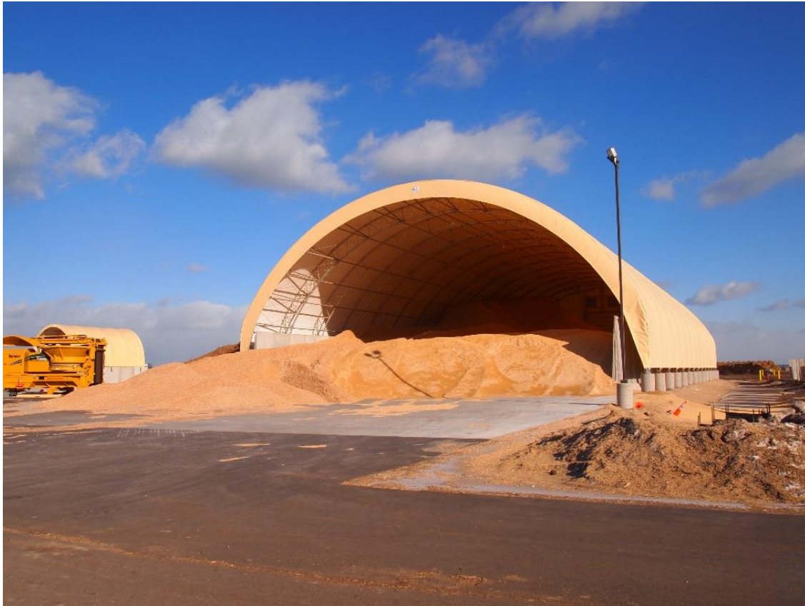
Biomass staging facility, Koda Energy, Shakopee, MN
